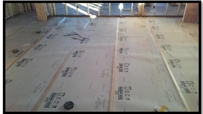
floor from inevitable messes expected to be made in the process of insulating, drywalling, painting and the routine worker muddy boots in and out of the house. A rolled heavy-duty cardboard (Ramboard) was laid down by the homeowners over the entire concrete slab, including the garage... so far, the product is doing its job!
