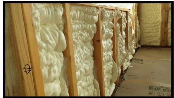
insulation that also has excellent sound deadening qualities. This two-part approach, also termed “flash and fill”, results in a highly insulated wall system (R-21 cavity insulation, not including the exterior rigid insulation soon to be
