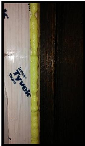
entry door that was installed. Local craftsman [Keith Mion](#) assisted the homeowner in these door installation efforts. After these installations, the homeowner further enhanced the home’s air tightness by sealing the gaps around windows and exterior doors with low-expanding foam and/or caulk. Elimination of air leakage will lead to a more comfortable and energy efficient home.
